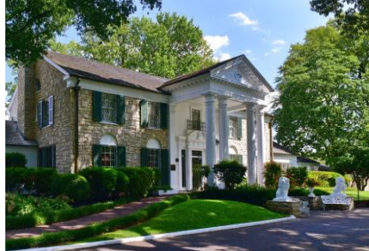
Exterior of Graceland mansion ©Memphis Travel
